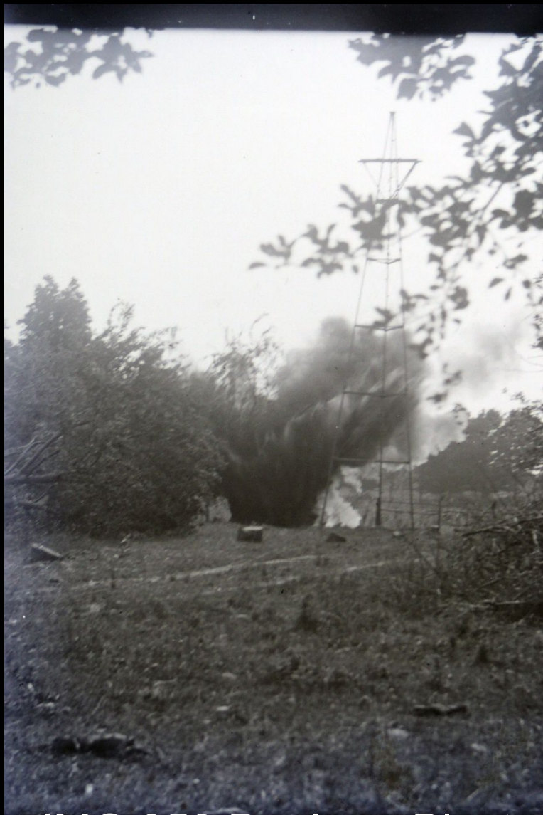
IMG 359 Dunlap - Blast on Powerline, Plate #166
